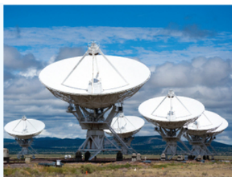
Figure 1.7.12: Energy reflects off of the parabolic reflector and is collected at the focal point. (credit: modification of CGP Grey, Wikimedia Commons)
